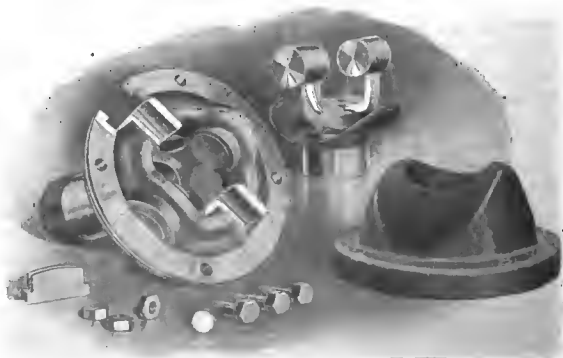
"Type C" Joint Dissembled, Showing the Parts.
